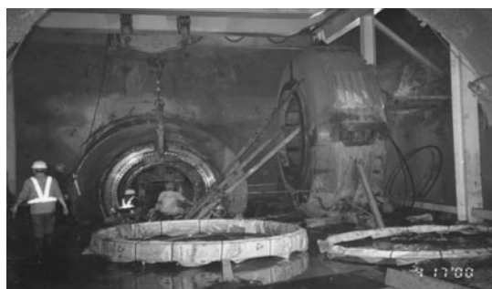
Fig.7 The first replacement of TBM ring gear
