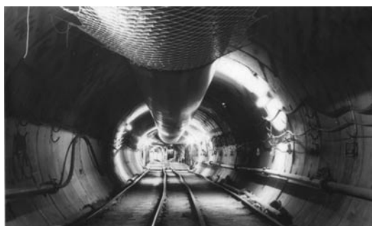
Fig.3 TBM back-up system & Pilot Tunnel
