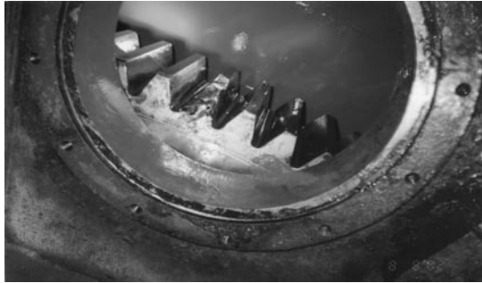
Fig.9 Two broken teeth on ring gear
