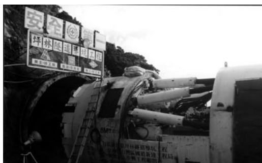
Fig.2 Final inspection of TBM before launching
